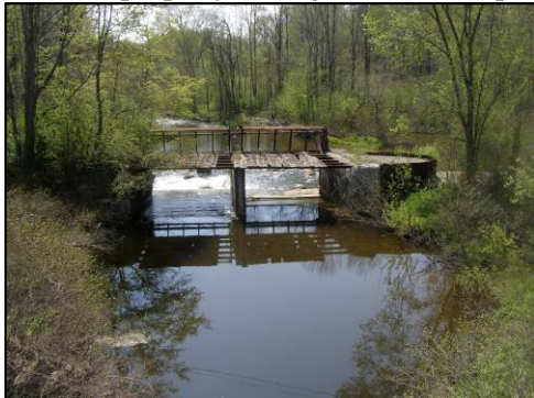
An abandoned dam located on Brokenstraw Creek near Jacquins, NY
