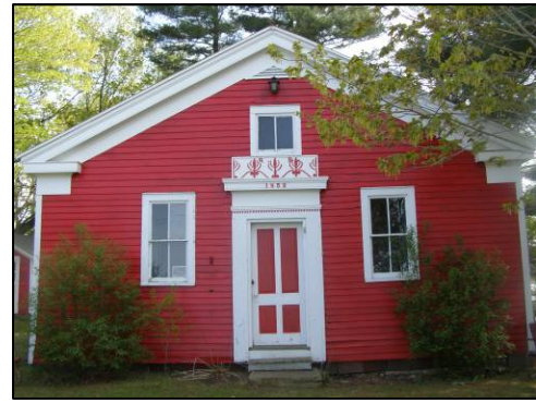
The Little Red School House in Clymer, NY
